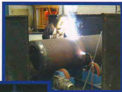
On-going welding on Bypass valve
