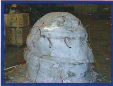
PWHT treatment going on
