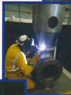
On-going welding of LP Bypass valve
